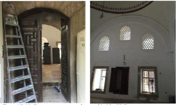
Figure 13,14. Classroom; entrance door and inside, 2015
