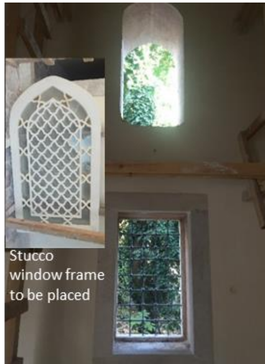
Figure 3.88. Original room window order, 2015
