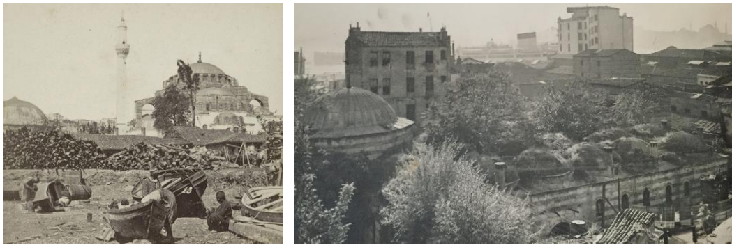
Figure 3.200. (left) Kılıç Ali Paşa Complex, photo by Sophus Williams, 1860's Figure 3.201. (right) Kılıç Ali Paşa Medrese from minaret, at the beginning of 20th century from Restoration Report (archive of KVKBK 1)
