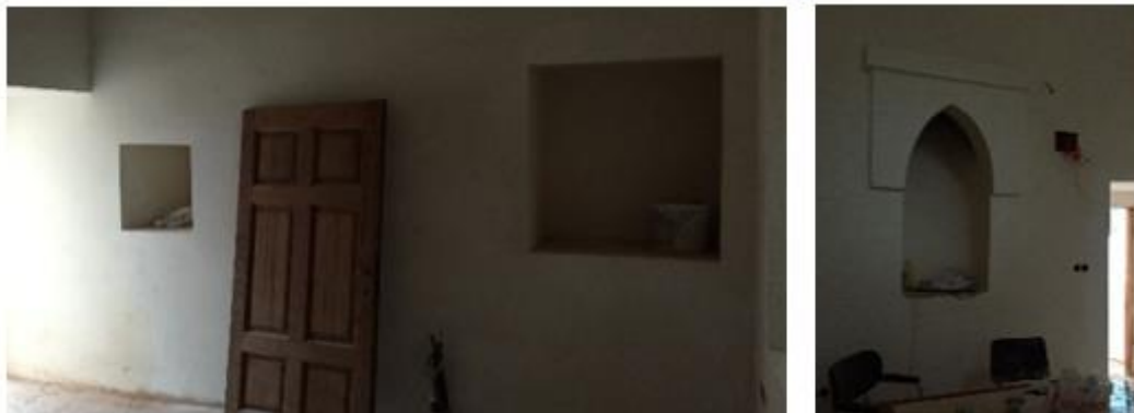
Figure 3.31. Original ground floor rooms' niches, and original fireplace, 2015
