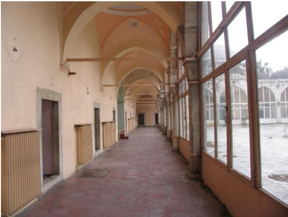
Figure 3.97. Metal framework addition and heating system intallation in 1960 closure of revaks of Şehzade Medrese (archive of DGF)
