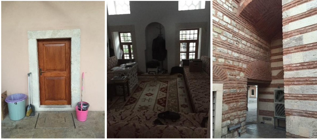
Figure 3.275. (left) Control cap on the installation channel surrounding revaks, 2015 Figure 3.276. (middle) The room refurnished for calligraphy workshop, 2015 Figure 3.277. (right) External airconditioning unit of the classroom, 2015
