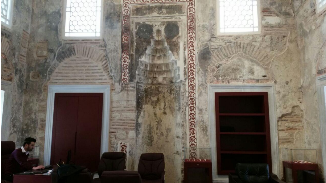
Figure 4.15. Use of the classroom of Siyavuş Paşa Medrese as administration office in 2015
