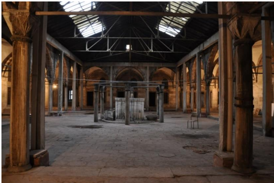
Figure 3.300. Courtyard of Sultan Ahmet Medrese in 2011, before restoration
