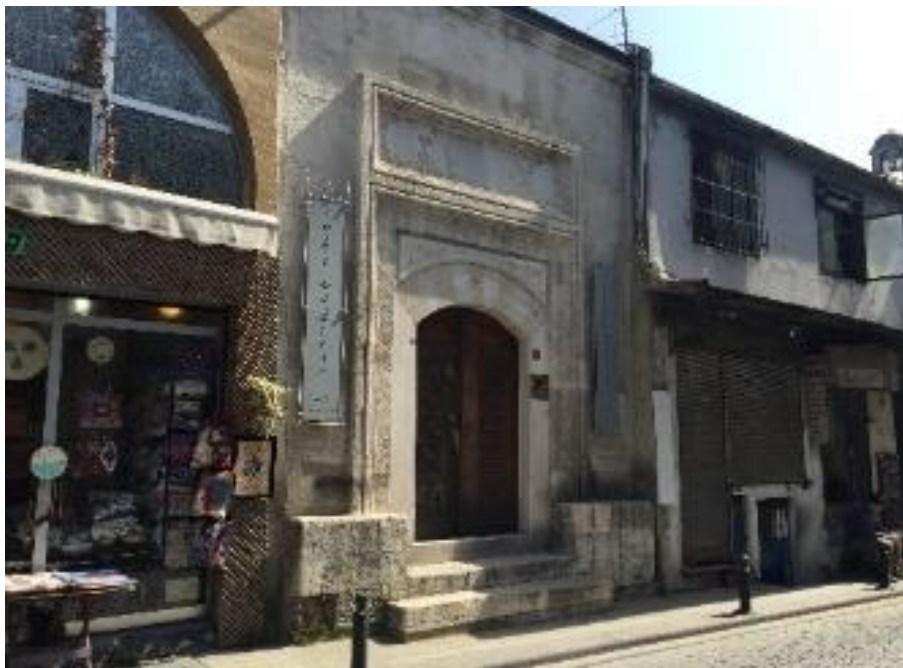
Figure 3.161. The main entrance, 2016
