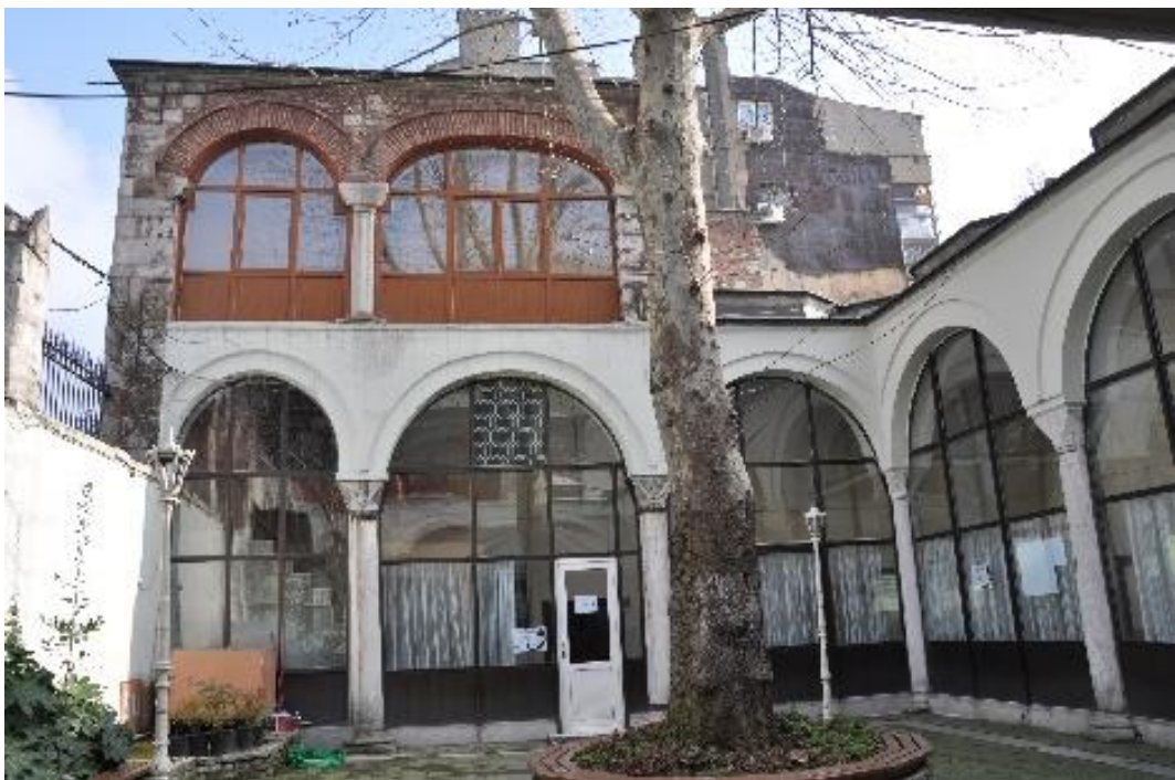
Figure 3.39. Courtyard and revaks in 2011
