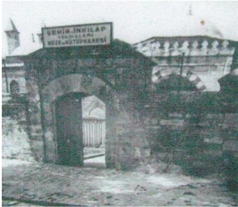
Figure 3.20. Beyazıt Medrese and original garden walls before demolishing in 1950's (archive of Yılmaz Yapı)
