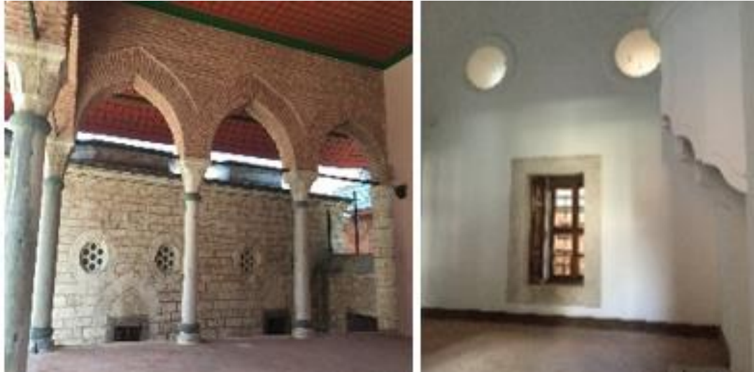
Figure 3.69. South-west room's windows from west (from outside) and inside, 2015
