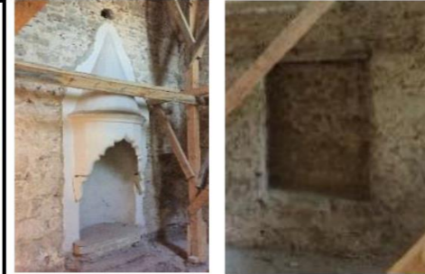
Figure 11,12. Fireplace and medium niche in room, 2015
