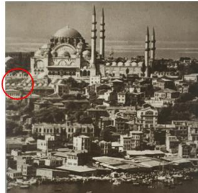
Figure 3.154. Süleymaniye Complex and Rabi Medrese from Galata Tower in 19th century. (Fatih Conservation Plan Report 2003)
