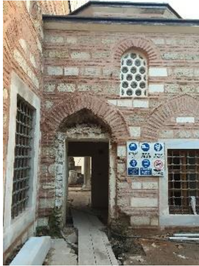
Figure 3.38. Window alteration in the room next to the classroom after 1975 interventions in unknown date, 2015
