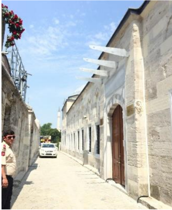
Figure 3.316. Main entrance and a steel made construction fixed to the facade for a shelter, 2015
