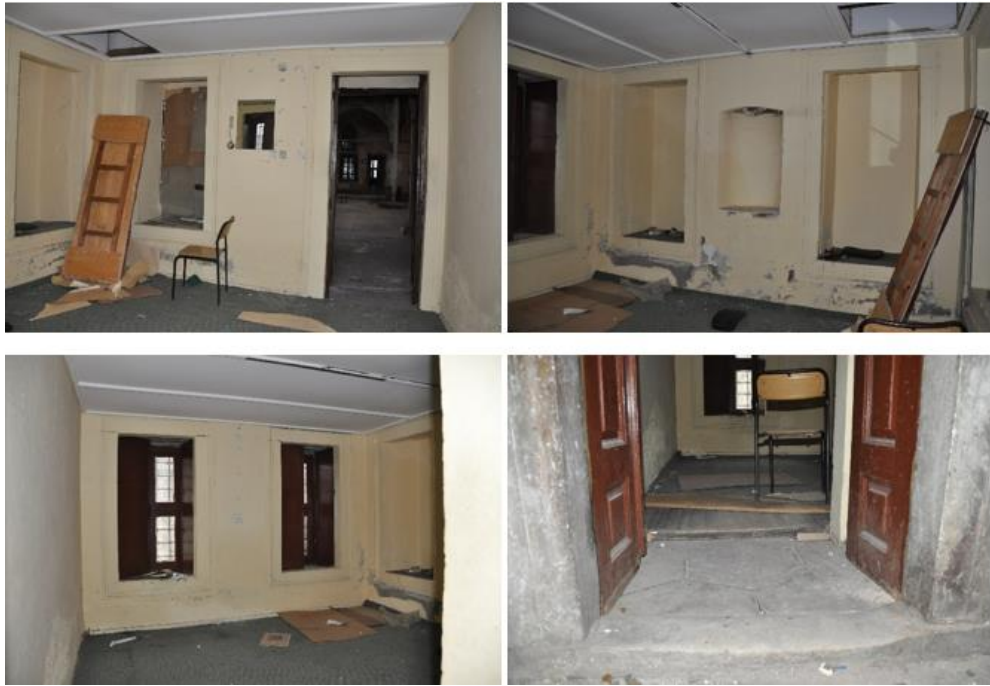
Figure 3.301. The situation of unpermitted past interventions in the room on south west side of the entrance eivan of Sultan Ahmet Medrese in 2011, before restoration
