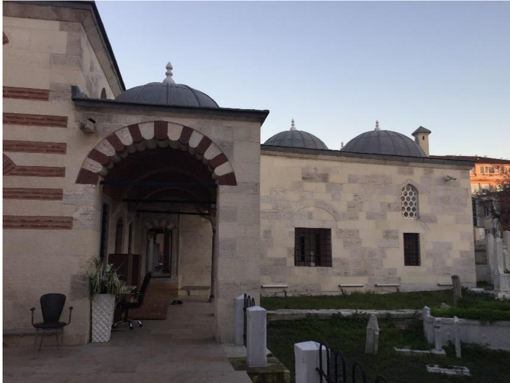
Figure 3.267. Revaks of the classroom from west and the entrance of the medrese at the end, 2015
