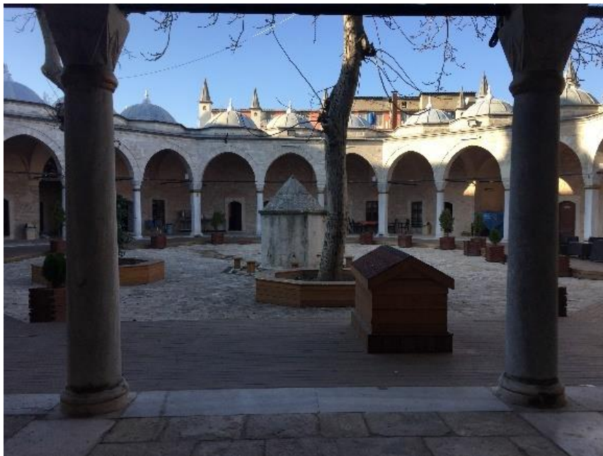
Figure 3.140. View of courtyard from entrance eivan, 2015
