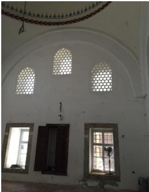
Figure 3.13. (Left). Classroom; entrance door and inside, 2015
