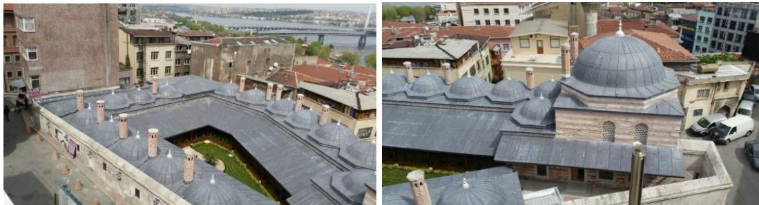
Figure 3.235. (left) General view from South East, 2016.
