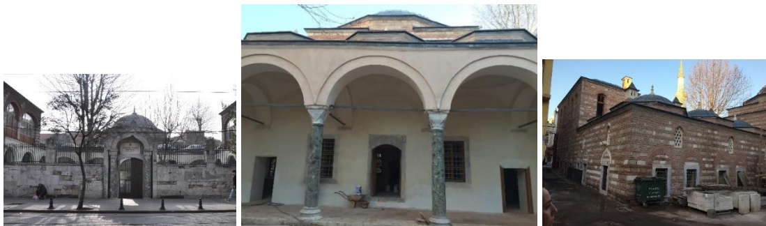
Figure 3.27. (left) Main entrance and courtyard, 2011 (before restoration)
