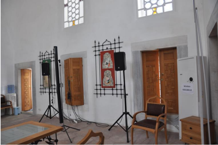
Figure 4.8. Broadcasting and air-conditioning installations in the classroom of Rabi Medrese in 2015
