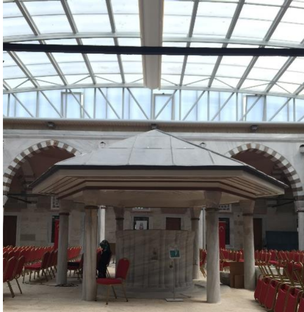
Figure 3.309. Courtyard roofing and reconstructed fountain roof, 2015
