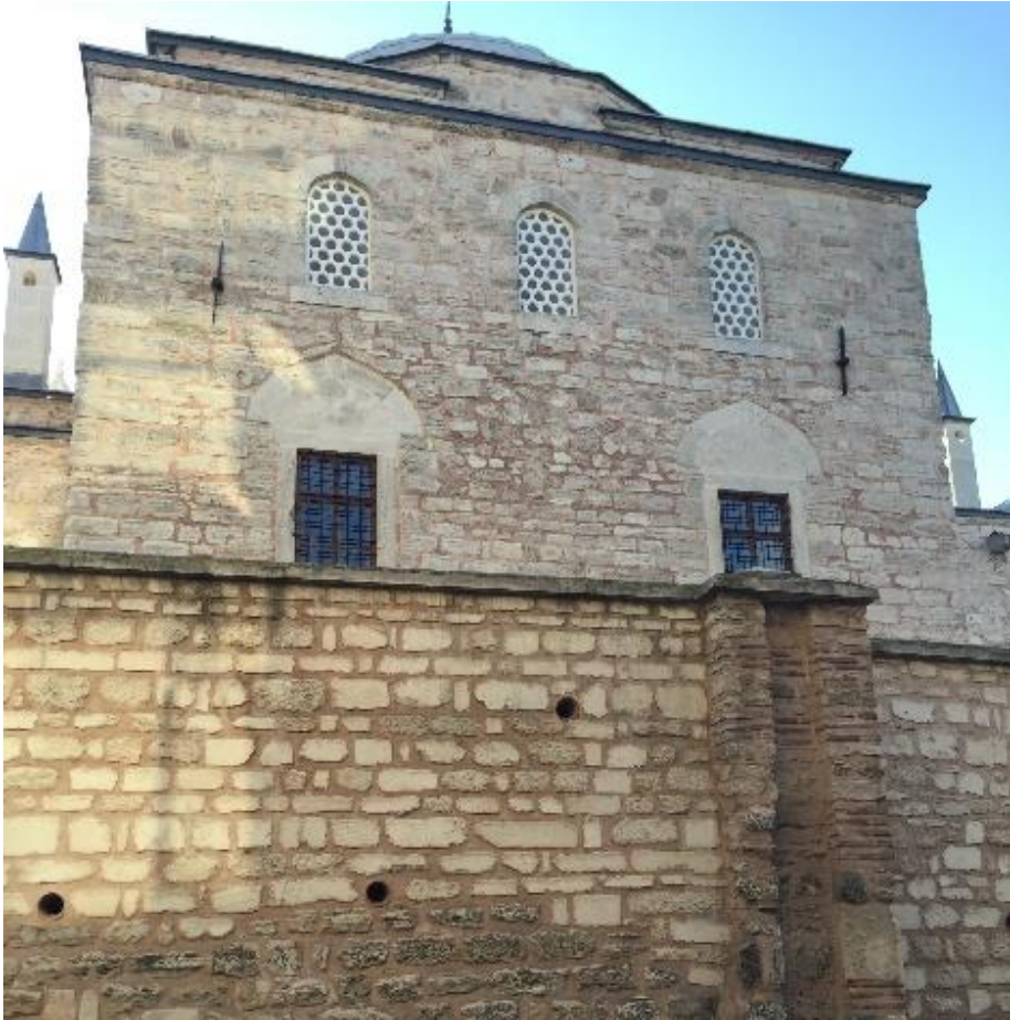
Figure 3.125. Classroom from north east, 2015
