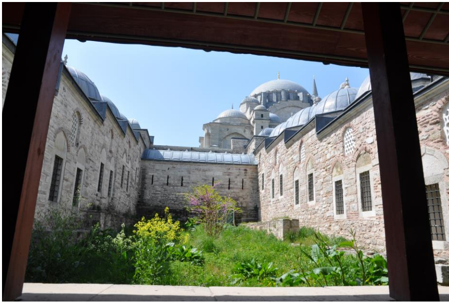
Figure 3.165. Outer façade and window order of the rooms in Rabi and Salis medreses, 2016
