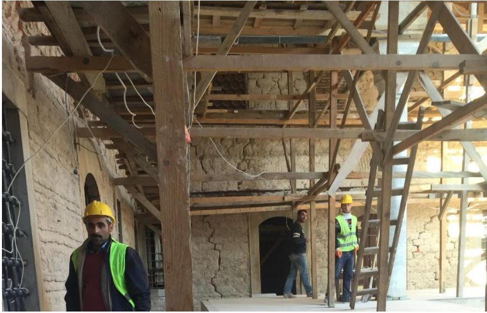
Figure 2.34. Structural cracks on Tabhane Medrese in Fatih Complex. 2016
