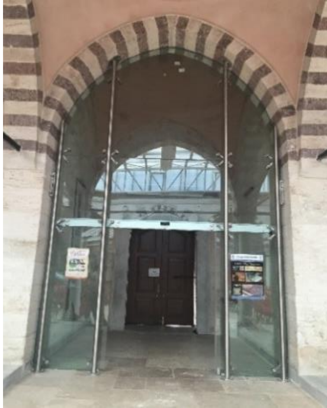
Figure 3.311. Glass separation of entrance eivan on revaks side, 2015
