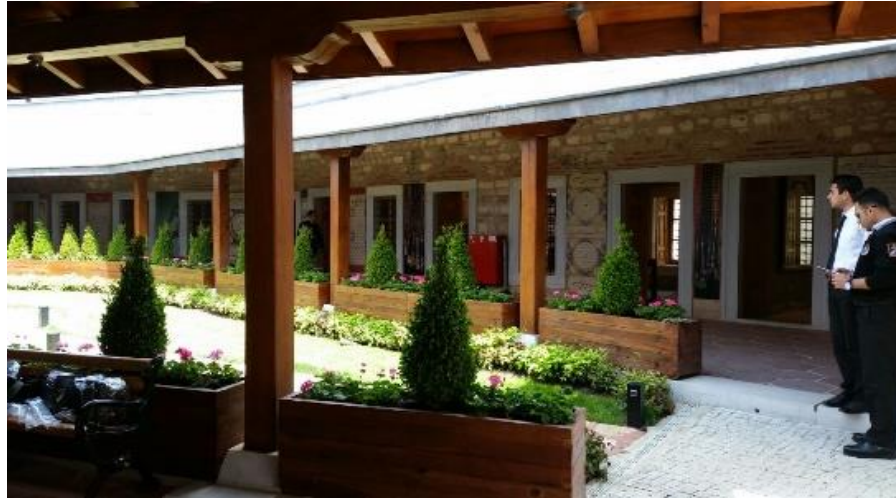
Figure 3.250. Courtyard and revaks from South, 2016.
