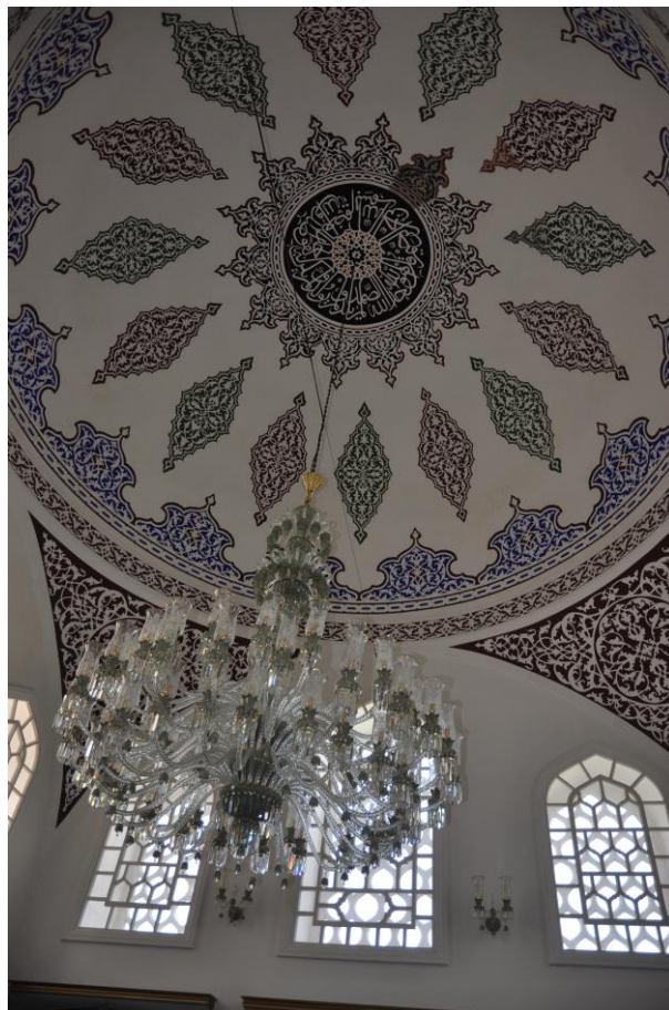
Figure 4.25. Ornamented architectural elements in the classroom of Sultan Ahmet Medrese in 2016
