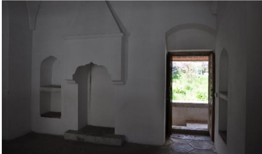
Figure 3.167. Interior of a typical room
